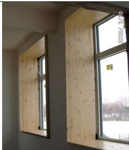
Figure 26 Window frames from the inside
