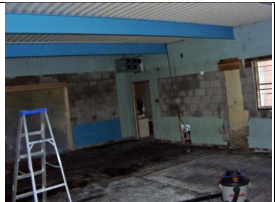
Figure 2 Inside of schoolhouse early in renovation
