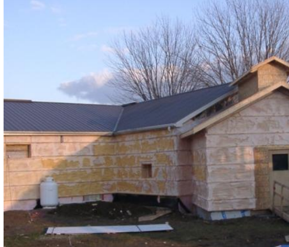
Figure 9 Polyurethane foam insulation filling Larsen Truss
