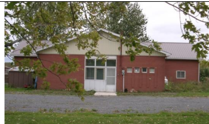
Figure 1 The schoolhouse before renovation
