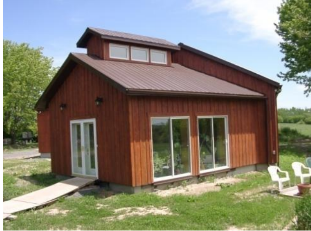
Figure 3 The new addition -- a combined solarium/mudroom
