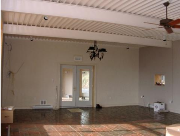
Figure 11 Original steel ceiling, stucco walls, and paver floors
