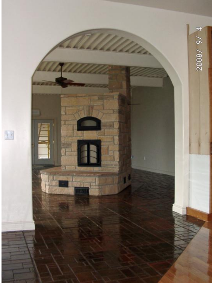
Figure 22 Finished paver floor and oak floor.
