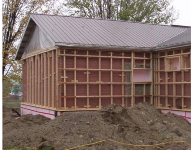
Figure 8 Building the Larsen Truss
