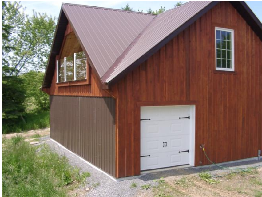
Figure 27 Garage with provisions for solar air heating collector
