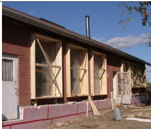
Figure 25 Deep window frames to accommodate Larsen Truss
