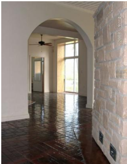
Figure 10 Painted stucco over block walls and floor pavers
