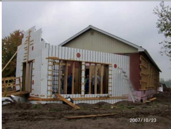
Figure 14 Mudroom/Solarium ICF walls
